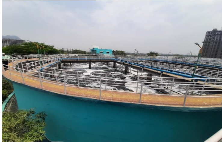
SBR at STP Mumbra Thane Municipal Corporation
