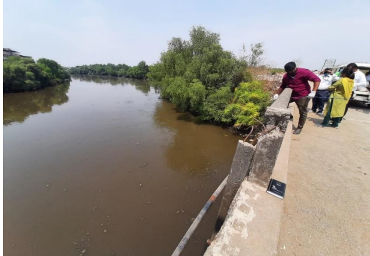
Desai Creek down Stream, Chuha Bridge, Diva (High Tide)
